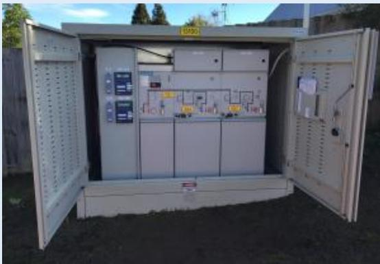
Figure 11. Bosecker Class B with automated switchgear.
