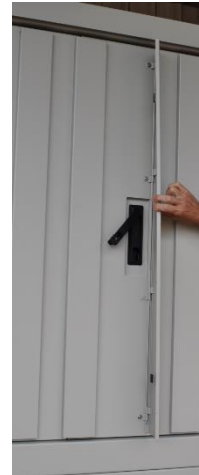
Figure 5. External locking mechanism.
