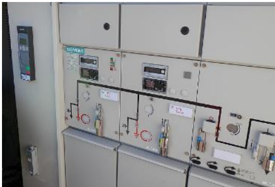
Figure 10. SIPROTEC 7SJ80 automation and 8DJH 'RRL' configuration.
